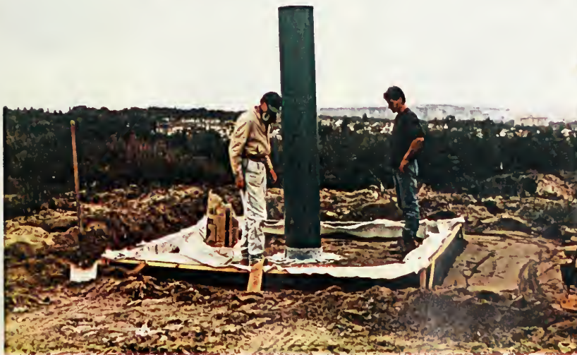
A 15: FINAL SAND LAYER APPLIED. PERIMETER OF MONITORING WELL SEALED
